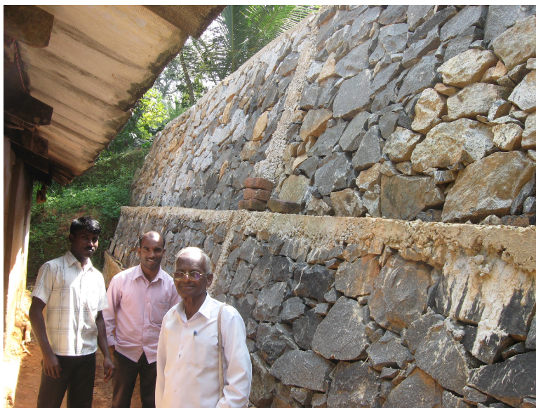
A congregational member, Mr. Shermar and Rev. Dr. Victor stand beside the retaining wall built by MMS at Emmanuel Lutheran Church in Mundakutty
